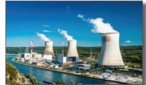
Cooling water control for power plants
