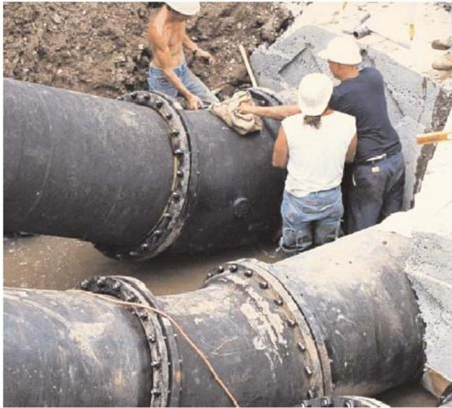
Ductile Iron pipe is often used for inverted siphons in difficult installations such as the stream crossing shown
